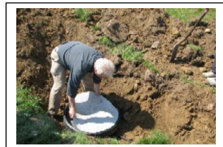
Installing Lysimeter - May 2007
